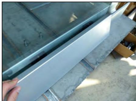
The Rail covers are pre-fitted with 3M tape. Cut Cover to size allowing for any corners or mitred cut outs. Please ensure main channel is clean and free from debris or grease.
