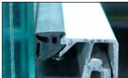
Press the seal into the gap between the glass and cover so that the small recess on the seal (which has a green stripe inside) overlaps the cover edge. Then, using your thumb or another device, move along seal until it's completely inserted. Please do not stretch seal too much whilst doing this as it will shrink back over time leaving a gap.
